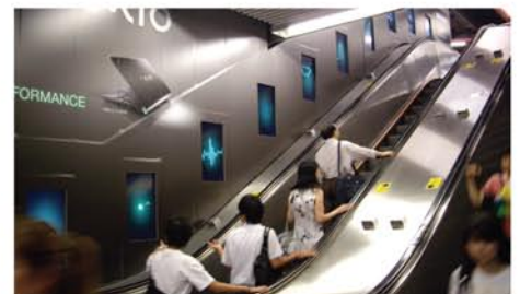
MTR JCDecaux installation Hongkong subway. Multi screen escalator setup.
