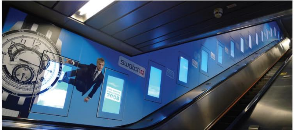
MTR JCDecaux installation Hongkong subway. Multi screen escalator setup.
